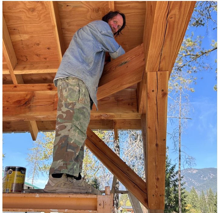
Handyman Jim Schulz climbs to new heights as he stains the wood on the Grange's new pavilion. Early October weather provided him perfect conditions.
